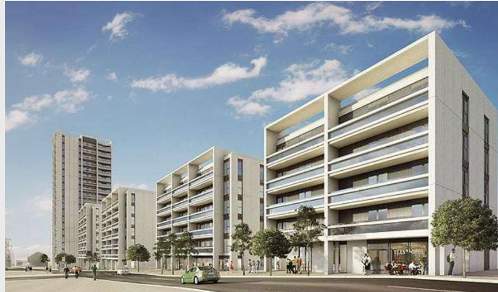
Above: Camden Council made its debut as a house builder, launching new homes for sale on the open market under its own name. Savills is marketing this development on behalf of the Council. The timing of development in Camden was interesting as the site was acquired during the economic downturn which provided a good opportunity to be more proactive during what was a quieter time in the market. However we note that it is becoming harder for the LA to continue to act as a developer due to rising costs and the comparative advantage that larger established developers and house builders enjoy .
